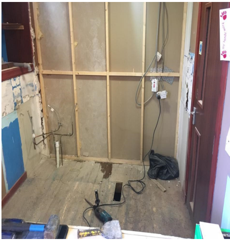
Construction is underway.
